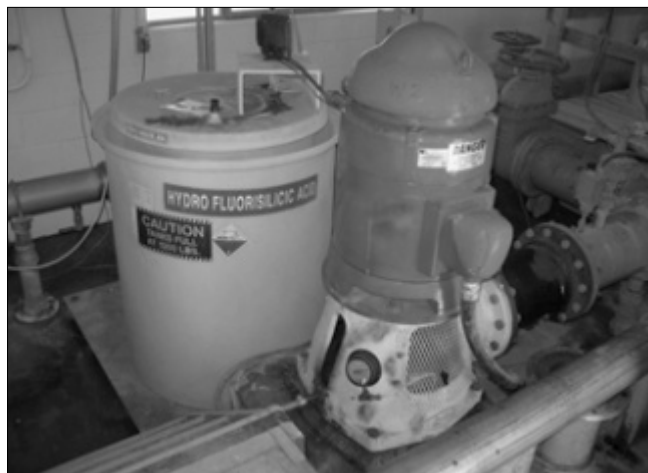
Hydrofluorosilicic acid tank and pump at the William Street pumping station in Waterloo, ON, prior to the 2010 referendum which led to the end of municipal fluoridation in the city.
